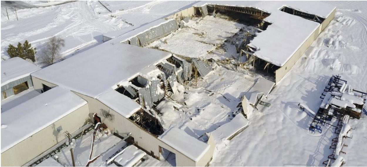
Last year a WOODsure client suffered a multi-million dollar collapse due to a combination of built up snow, and an unexpected mid-winter rain storm. The client then experienced several months of interruption to its operations as the entire plant required rebuilding. This same storm caused multiple large collapses for a variety of insurance companies in Eastern Canada before it subsided.
